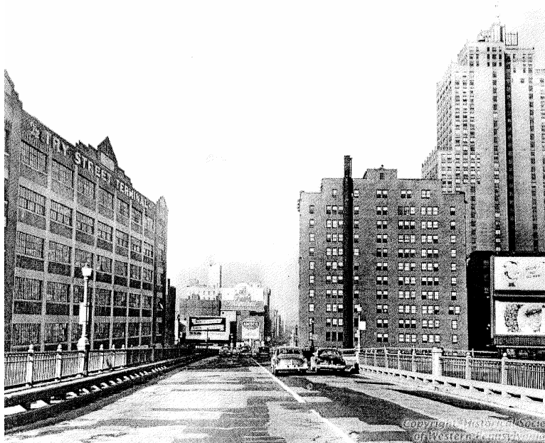
Figure 1.1-c The Try Street Terminal Building on left
